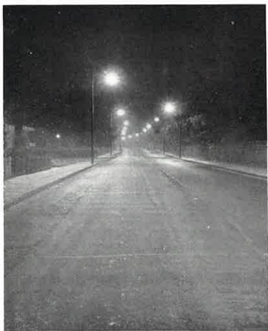
One of Britain's longest stretches of sodium streetlighting. Part of the new 7\frac{1}{2} miles stretch of Mazda lamps and lanterns on the Glasgow-Carlisle road.
