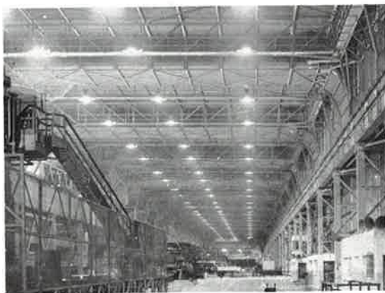
The Steel Company of Wales—the largest steelworks in Europe. Mazda lighting for the huge Rolling Mills includes over 1000 Blended Light Fittings designed for Mazda Tungsten and Mercury Vapour Lamps.
